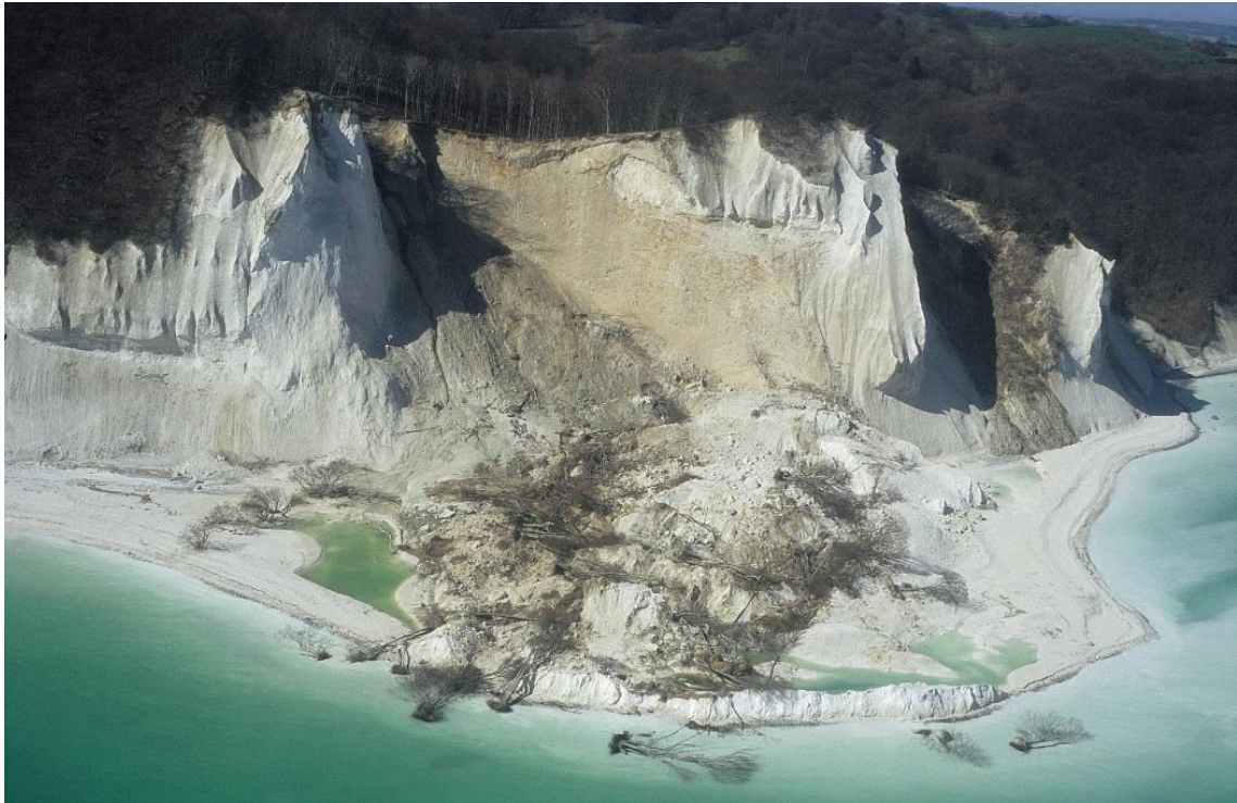
Figure 38. Example of landslide at Møns Klint, the Store Taler slide January 2007. More than 100.000 m 3 of chalk were displaced up to 300 meters away from the coastline.
